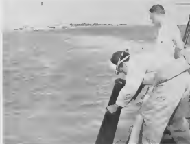
AS THE work boat moves past the intake, the rake pulls up sea grass. Moss from the grass had been clogging intake screens. Using a sight glass, below, a launch helper checks the cleared area.
